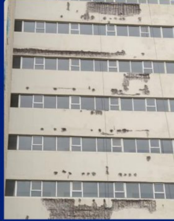
SPALLING REPAIRS
